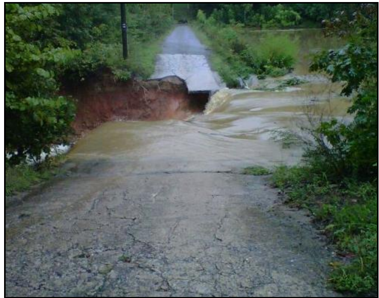
Heavy rains from a slow-moving system that came through the area on September 23, 2011 caused a breach in the Farmville Lake dam. The failure of the spillway took out a section of the road that passes over it. Source: T. Jordan Miles, III courtesy of Facebook
